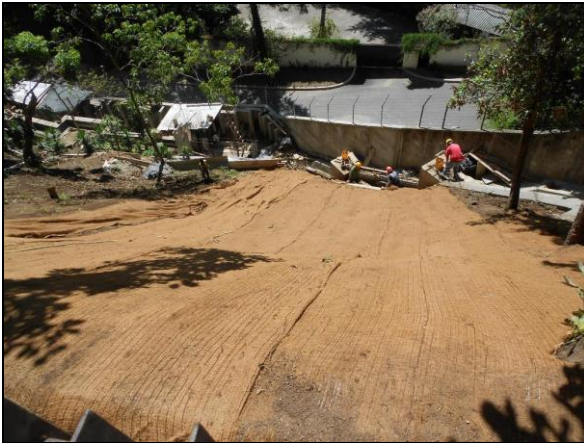
Photo 1: Biodegradable Geomat installed. Guatemala, May 2010.
