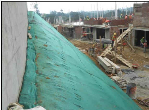
Photo 7: Synthetic geomat anchored to the slop. Antigua, July 2011
