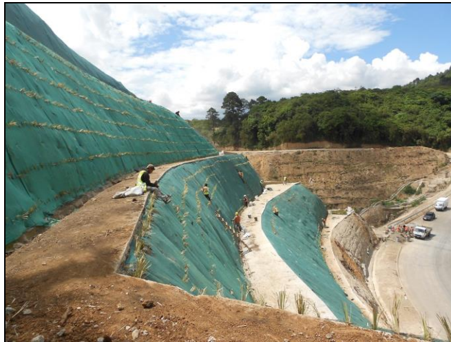
Image 9: Installation of the Vetiver System. Fraijanes, May 2013.
