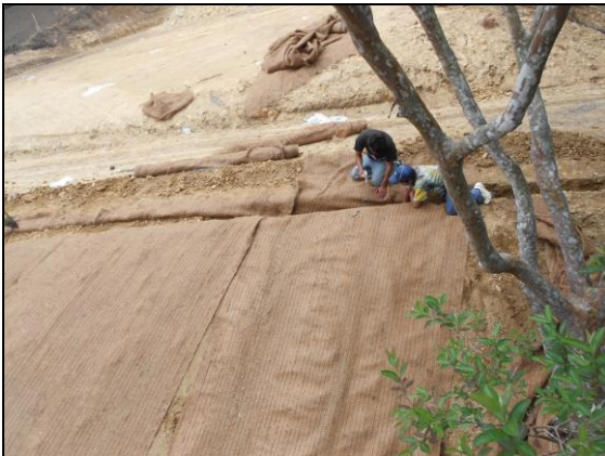
Photo 6: Anchoring ditch for the geomat. Quetzaltenango, December 2010
