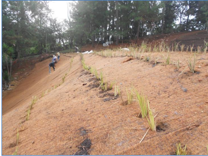
Photo 8: Installation of the Vetiver System. Cobán, June 2013
