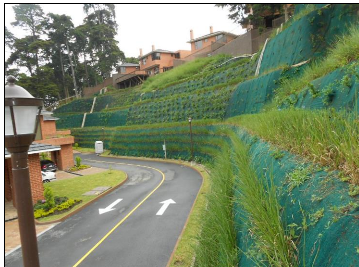
Photo 11: Slopes protected with geomats and the vetiver system. Concepción, June 2013
