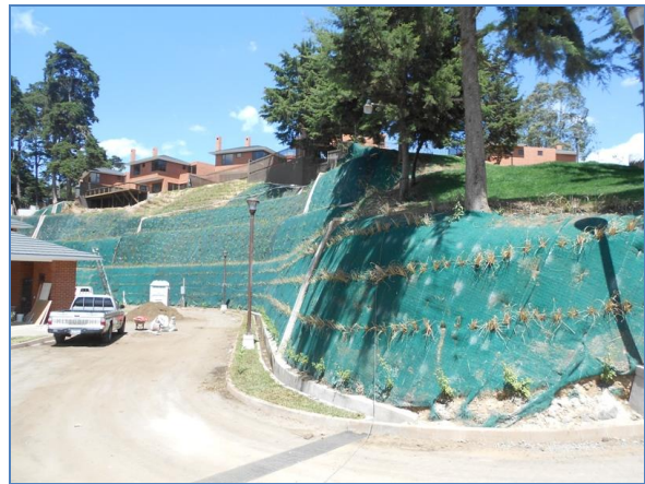
Photo 2: Synthetic Geomat installed. Concepción, February 2013.
